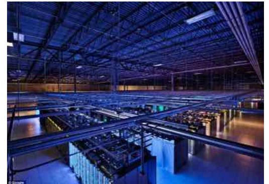
One of Google's dozen-plus server farms.
